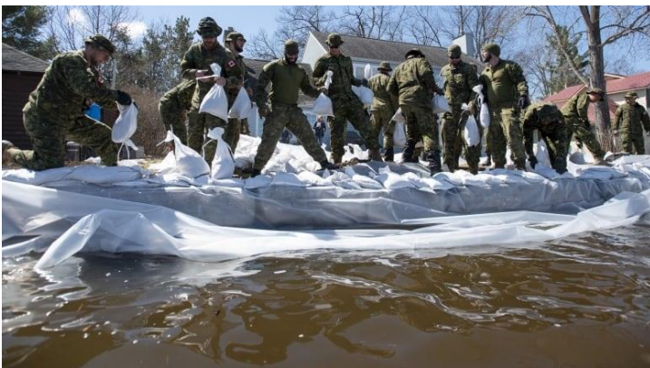
Troops build a wall of sandbags to protect a home from the flooding Ottawa River in Constance Bay, Ont., on Tuesday, April 30, 2019.
